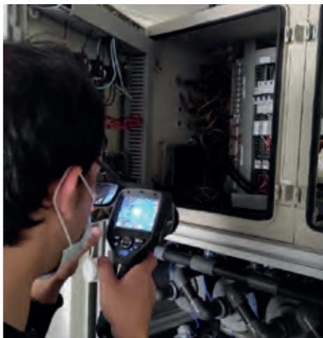
Infrared thermal imaging of the electrical cabinets of an ultra-filtration unit ©OiEau
